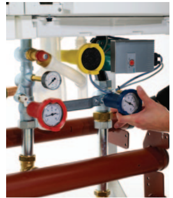
Step 4 Pump groups (additional accessory) and valves are connected to boilers and flow and return pipe work attached to the headers.
